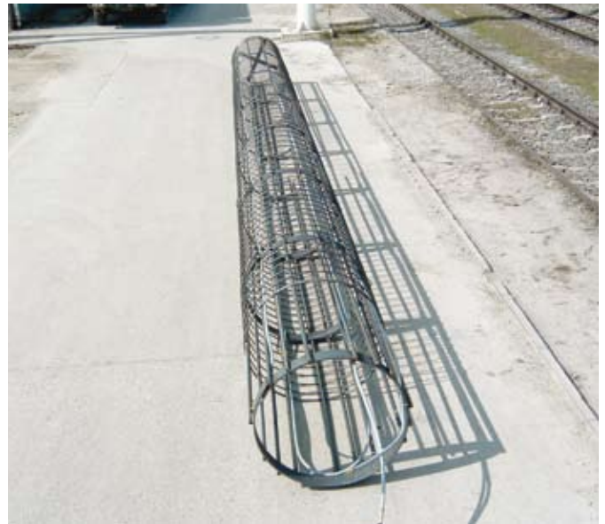
Fig. 14: Pilon energetic RAUGEO
