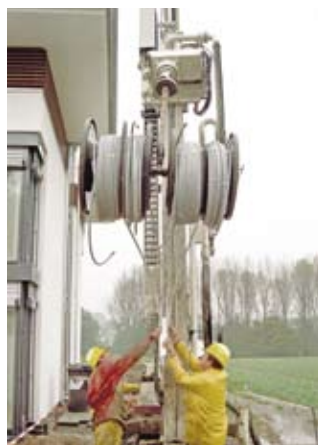
Fig. 4: Introducerea unei sonde RAUGEO PE-Xa
