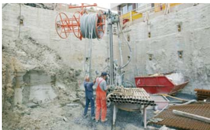
Fig. 52: Introducerea sondei
